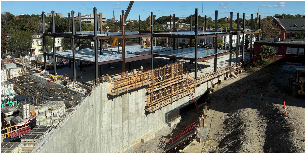
Structural steel progress, 10/02
