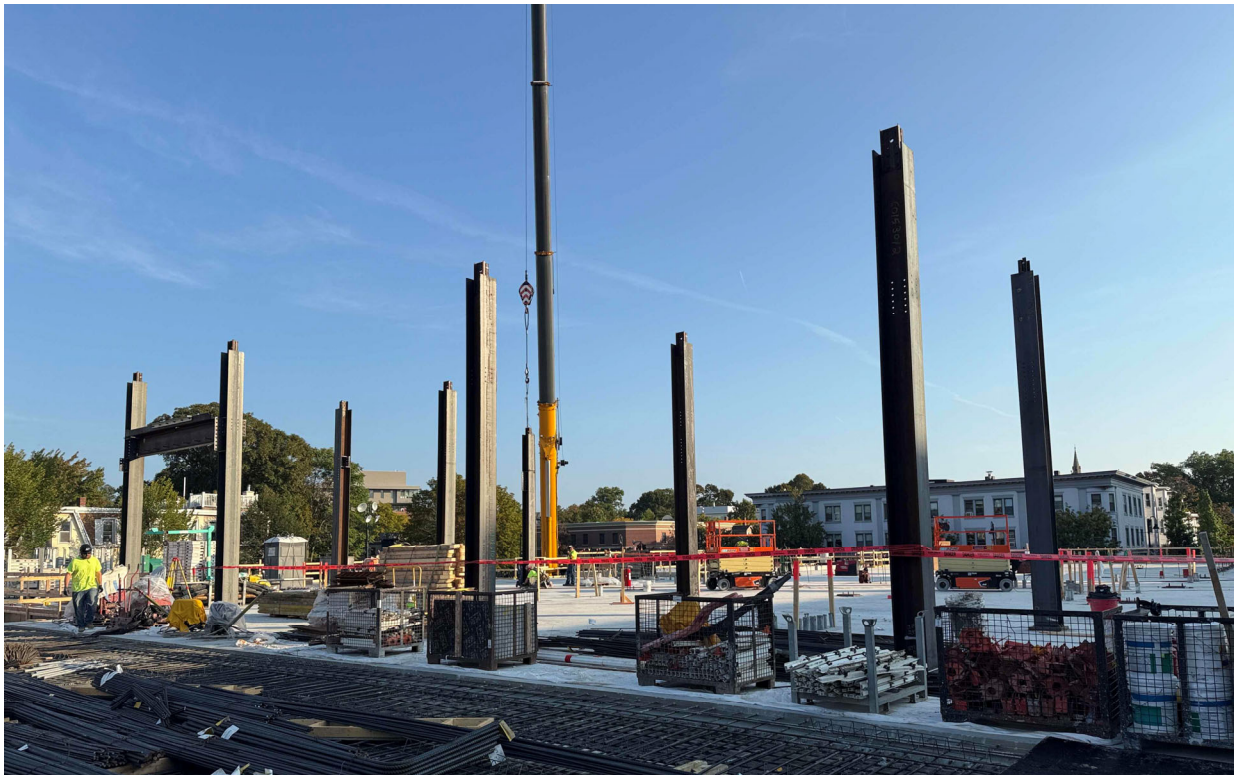
Steel erection begins, 09/23
