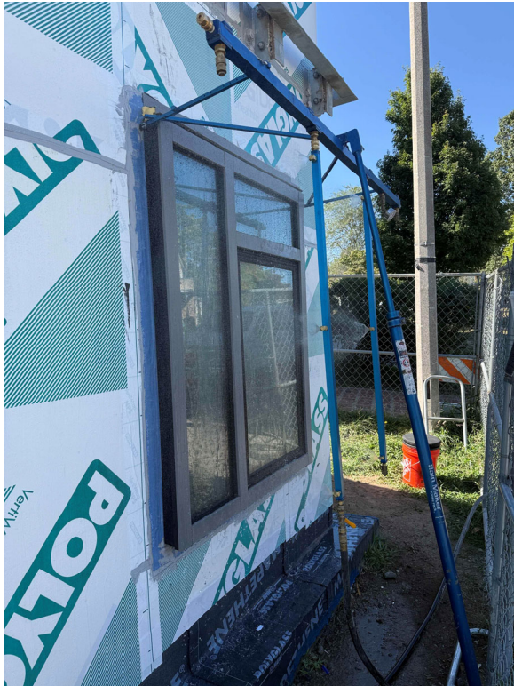
Window performance test @ mock-up, 09/03
