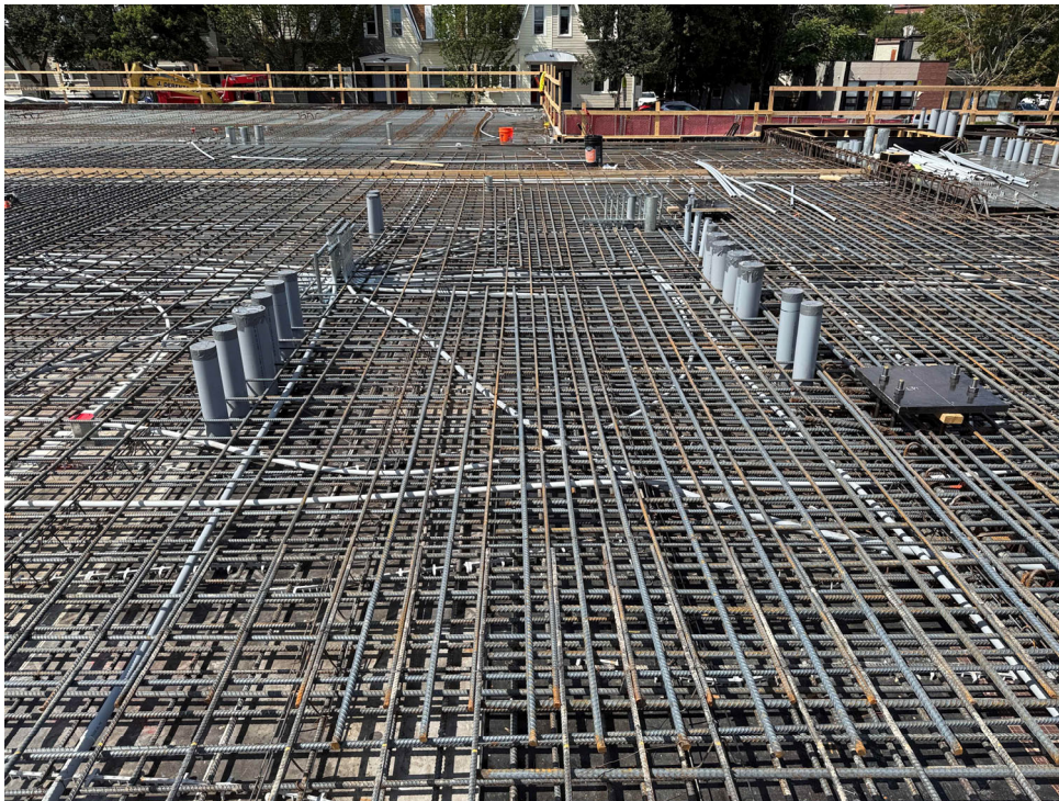
View of rebar and sleeves ahead of structural slab pour, 09/03
