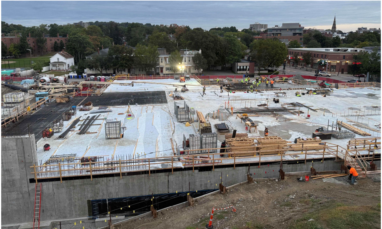
Overall structural slab post-pour, 09/10
