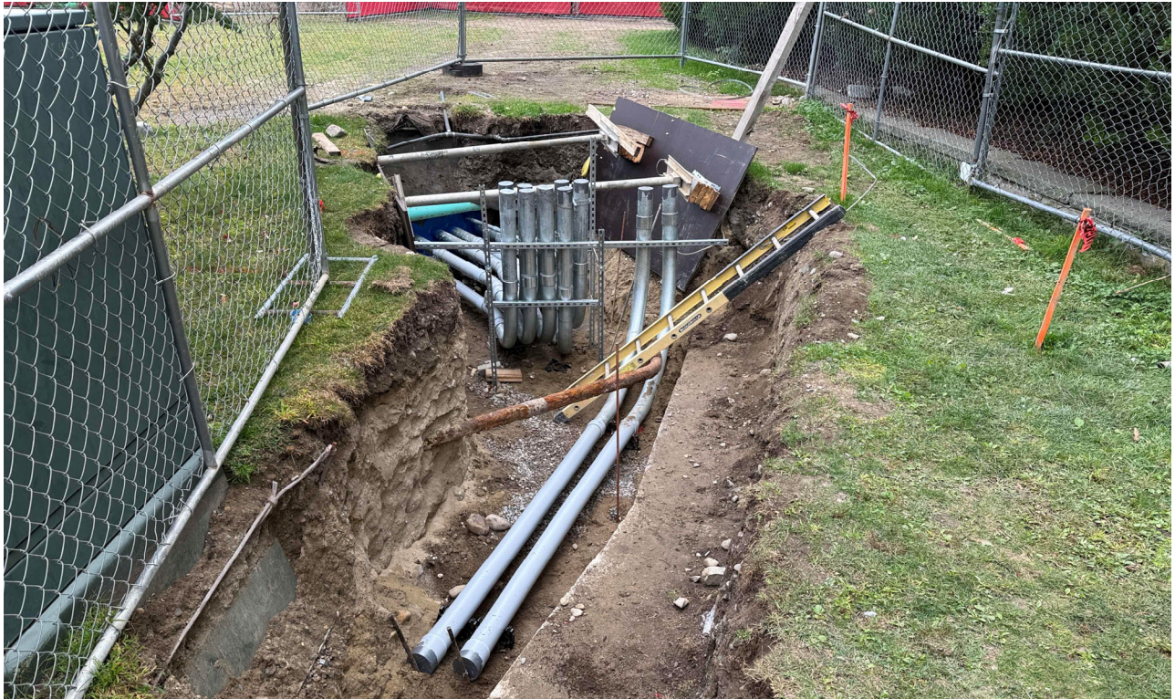
Conduit for transformer prepared for precast concrete pad, 09/24
