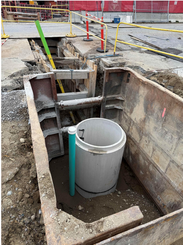
Site utilities run under School Street to new manhole structure, 09/05
