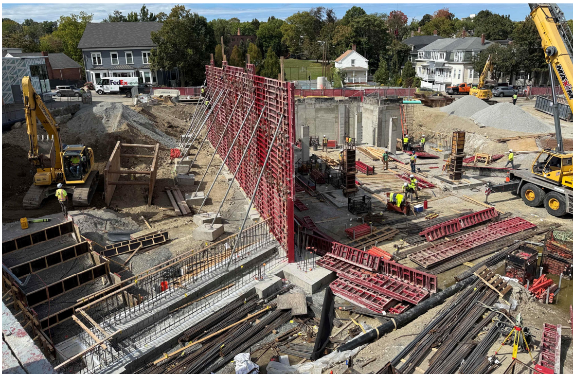
Formwork, rebar, foundation walls and concrete columns, Building B, 09/17
