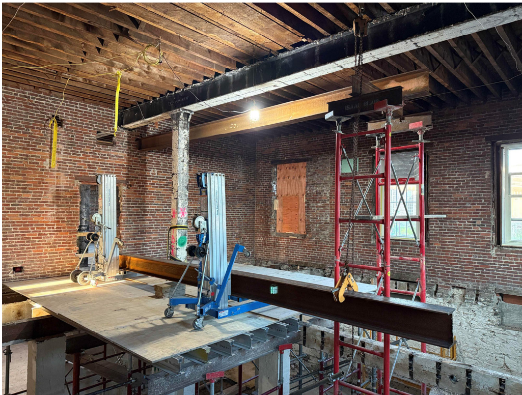
Shoring and inserting new structural beam in Historic Building, 09/09
