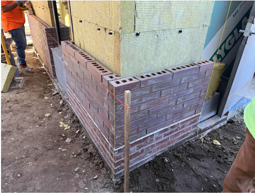
Brick underway at mock-up, 09/22
